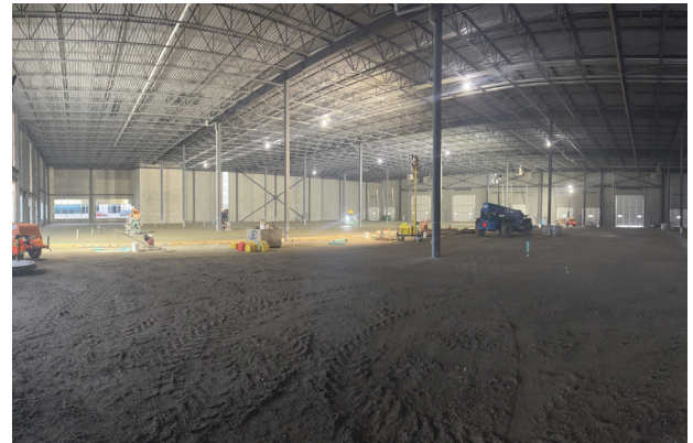
Though there is still a lot more work to be done before the new Food Distribution Centre can be opened, we are starting to see the dream become an actuality.
